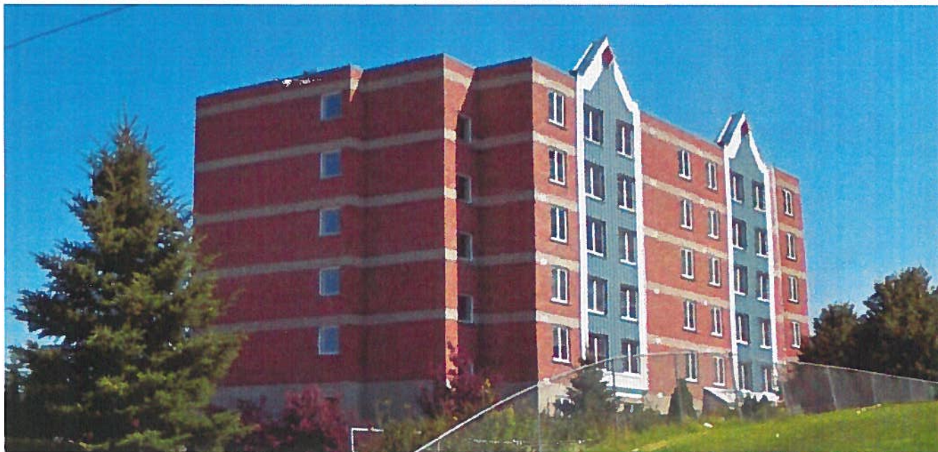
LE MIRAGE APARTMENTS 44 BORDEN AVENUE, TIMMINS, ONTARIO
